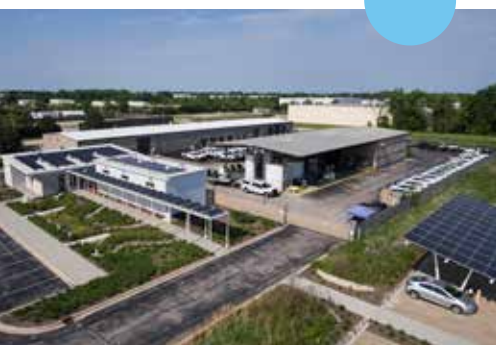
An aerial view of Clarke's Flourishing Garden location in Roselle, Illinois that recently became LEED Platinum certified.
